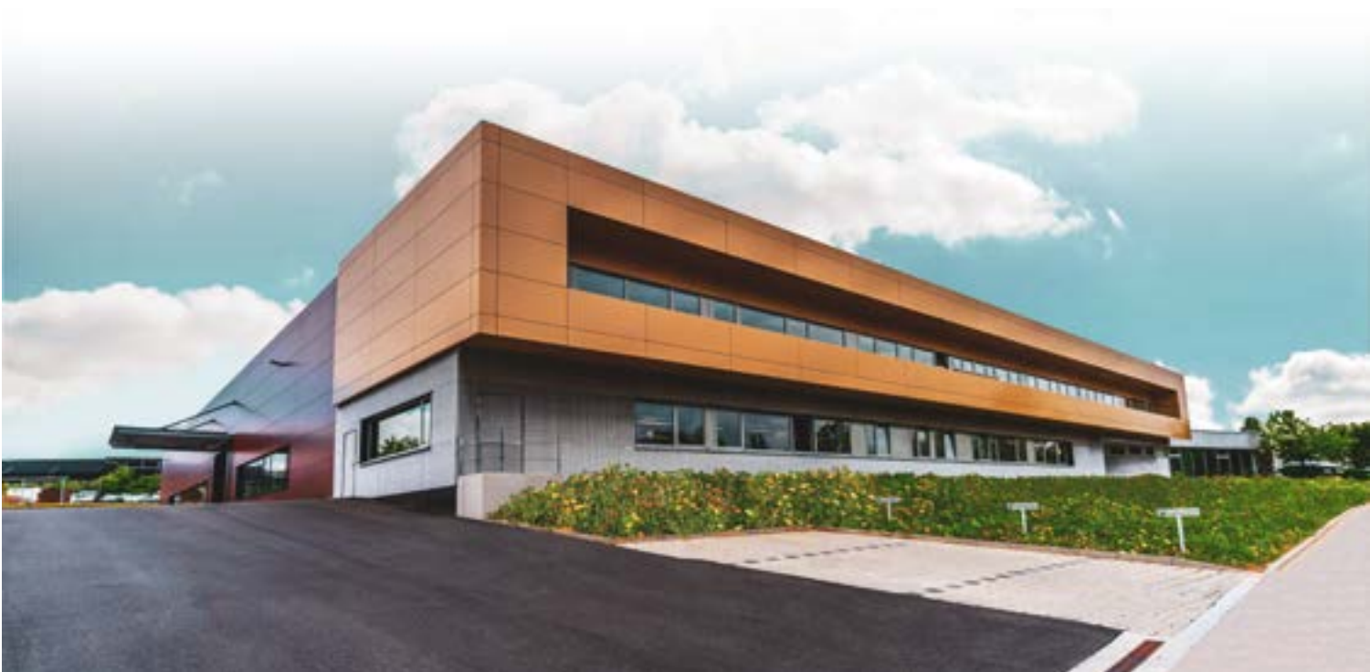
The head office of the syskomp Group in Amberg (Germany).
